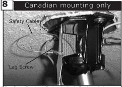
For Canadian installation in both flush and downrod mode the safety cable must be installed into the house structure beams using the 3" lag screws provided. Make sure that when the safety cable is fully extended the leadwires are longer than the cable and no stress is placed on the leadwires.
